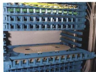
Splice and distribution modules can be inserted in and pulled out freely for operations.
